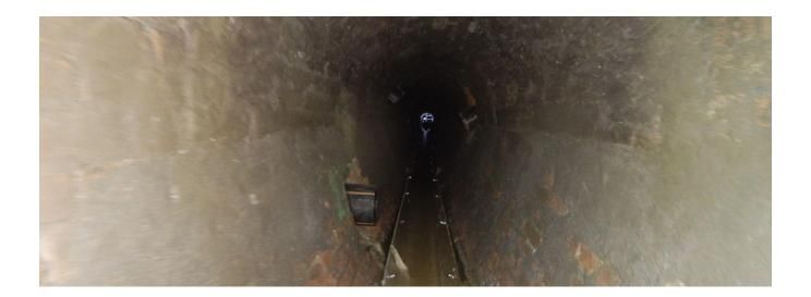
A narrow sewer tunnel was used for testing. This tunnel had curves, bends, and deviations in its trajectory after 20-30 meters. The only geometrical features in the straight sections were bricks or textured surfaces, manholes, and inlet/ outlet pipes.
